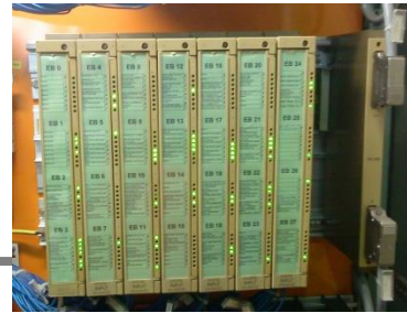
Expansion racks with digital input/output cards
