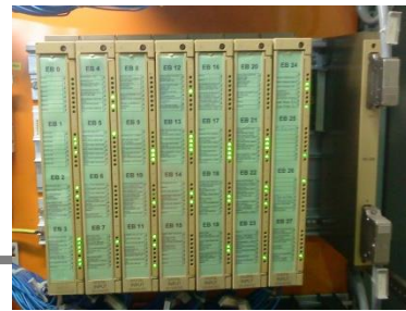
Expansion racks with digital input/output cards
